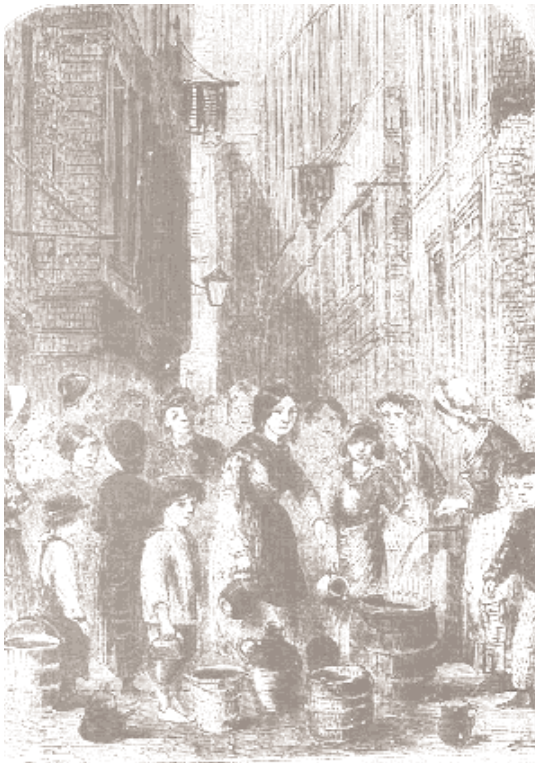
WATER SUPPLY—NO SUPPLY. FRYING PAN ALLEY, CLERKENWELL, LONDON.
